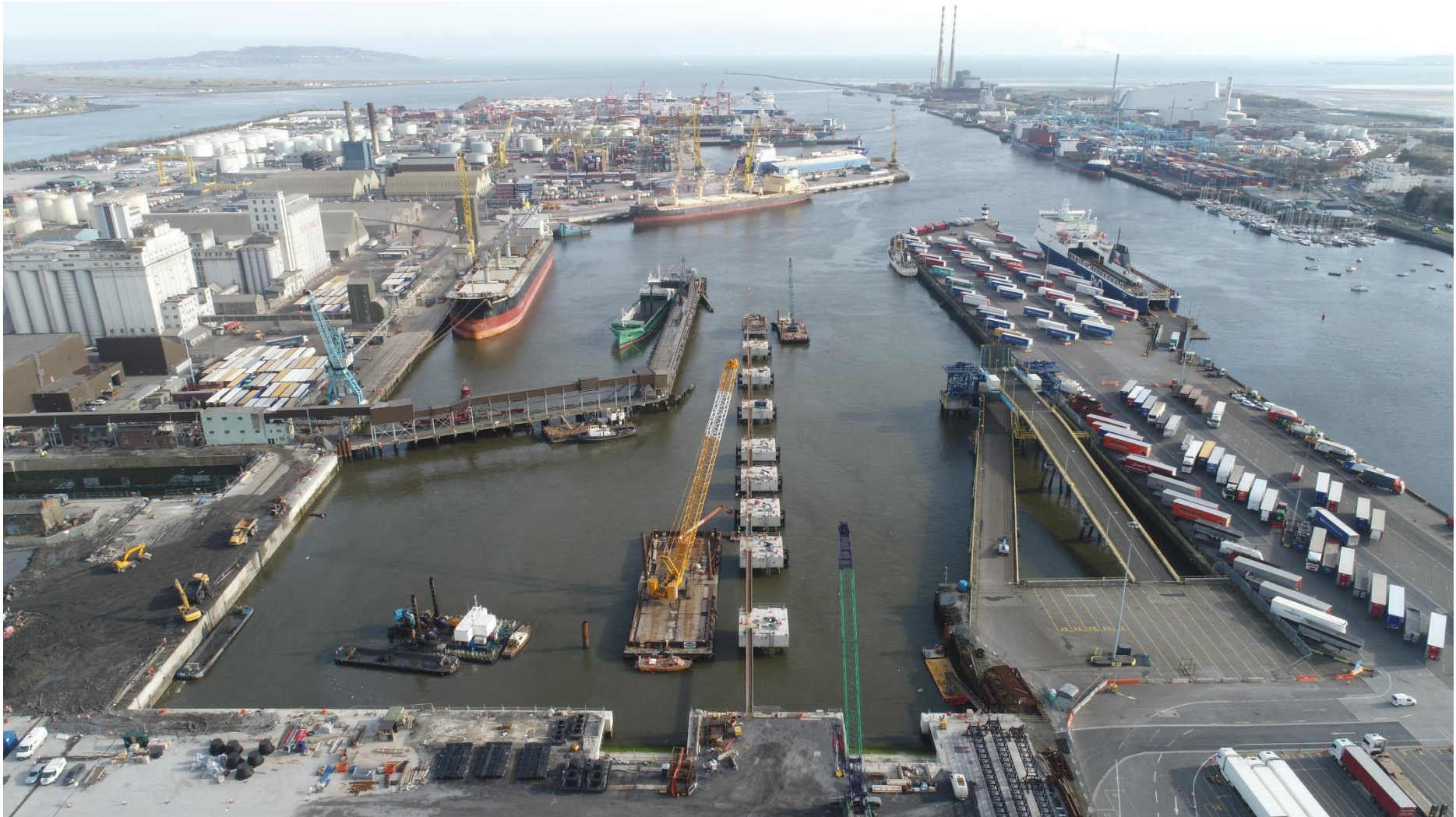
Figure 3: New Ro-Ro jetty for Seatruck under construction in Alexandra Basin
